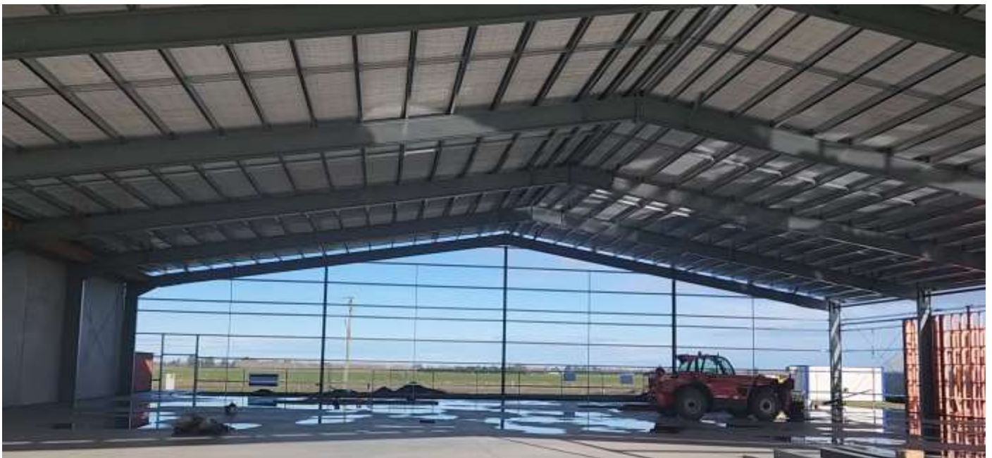
The new display hangar build as of late June this year.
